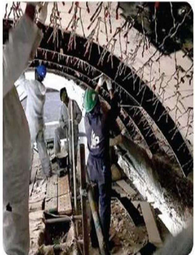
Refractory Lining Works at Kuwait Cement Company
