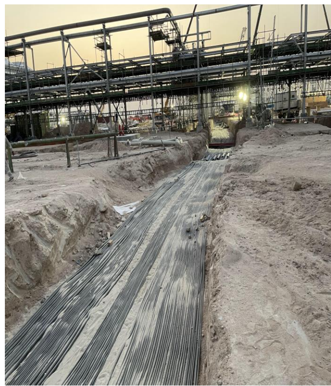
Power Cable Laying at JPF-5
