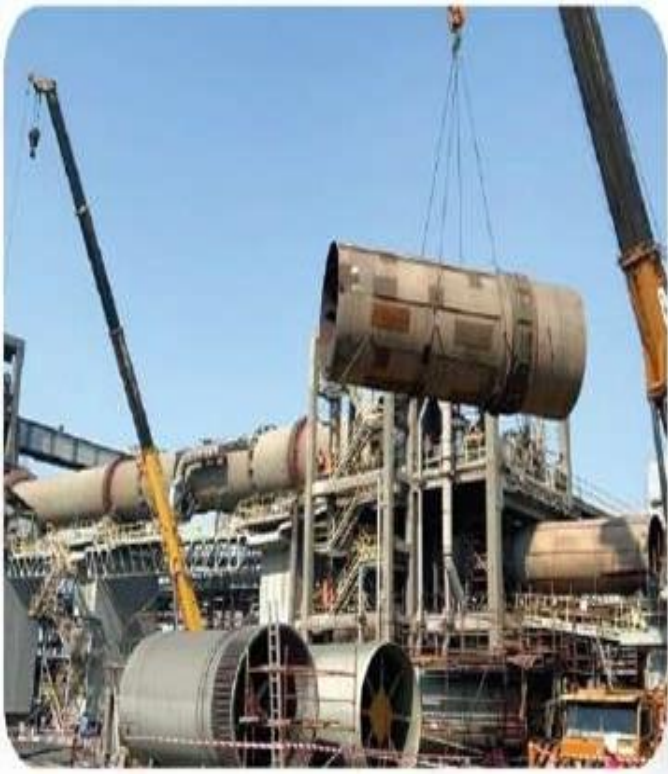
Erection of Cooler at PCIC
