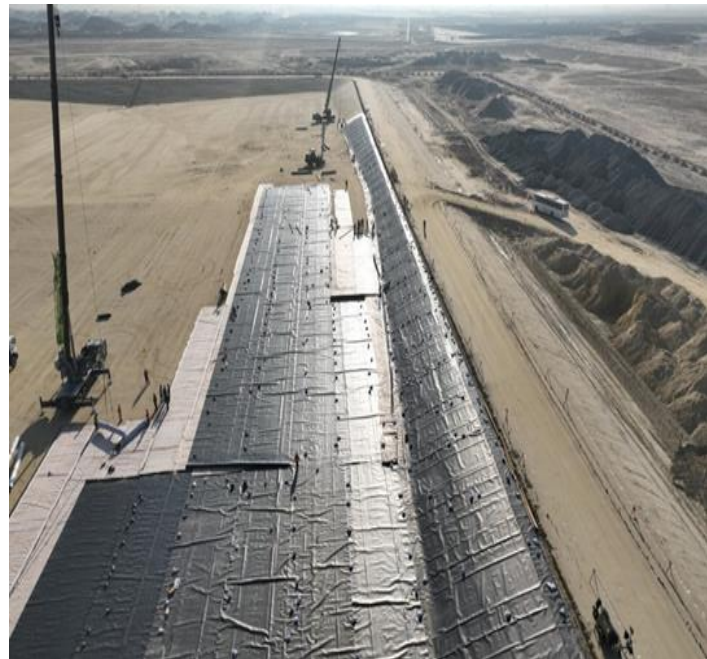
HDPE Lining work Soil Remediation Project
