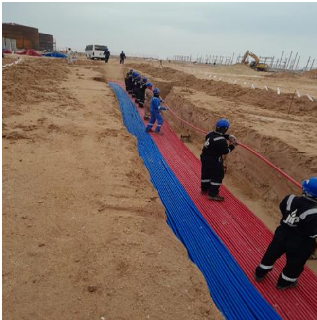
Instrument Cable Pulling at JPF5
