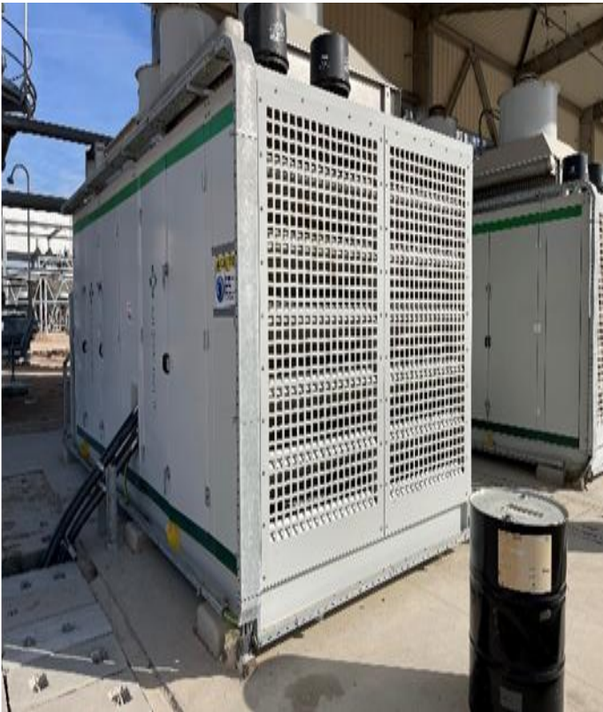
Air Compressor glanding and tray works at JPF-5.
