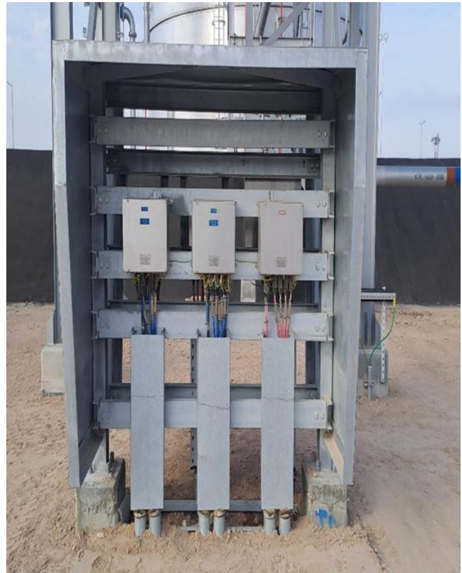
Instrument Junction Box Installation at JPF-5
