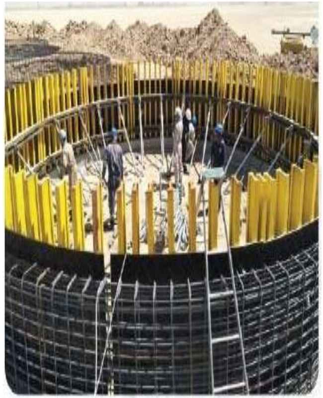
Tank Ring Foundation at JPF-4
