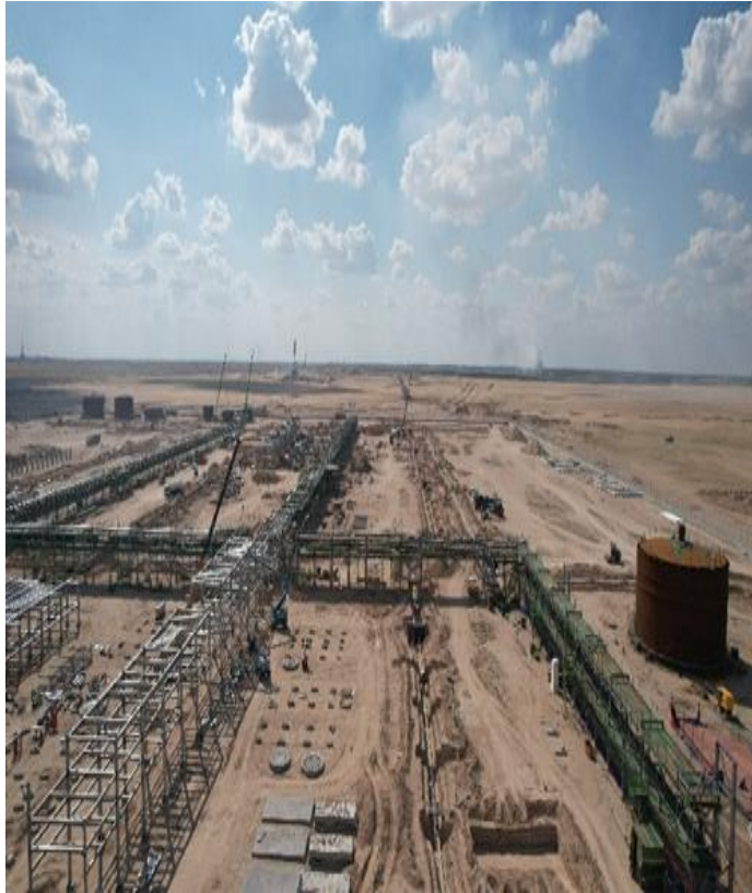
Pipe Rack Erection at JPF-5
