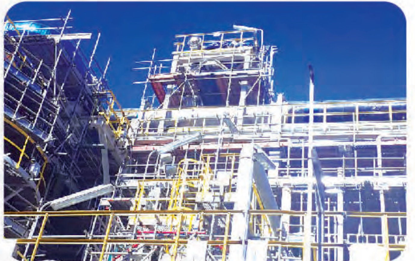
NRP - Scaffolding Project
